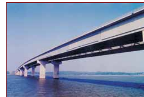
Lukens produced a great deal of structural steel for use in bridges.
